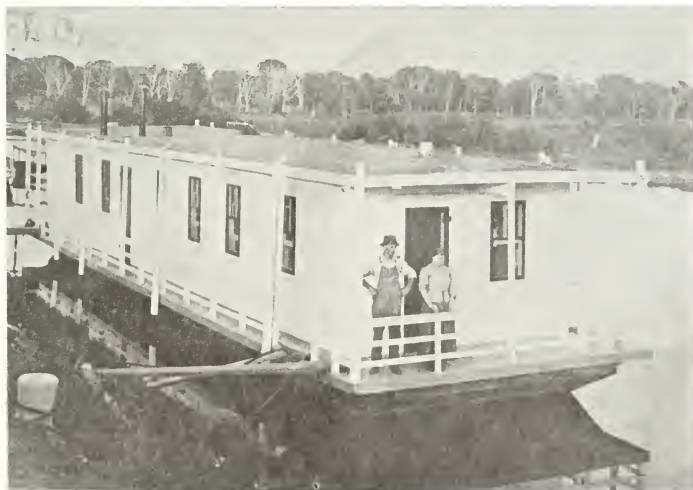
The Locktender's houseboat at Lock 1. (Photograph courtesy of Hennepin Canal Parkway.)
